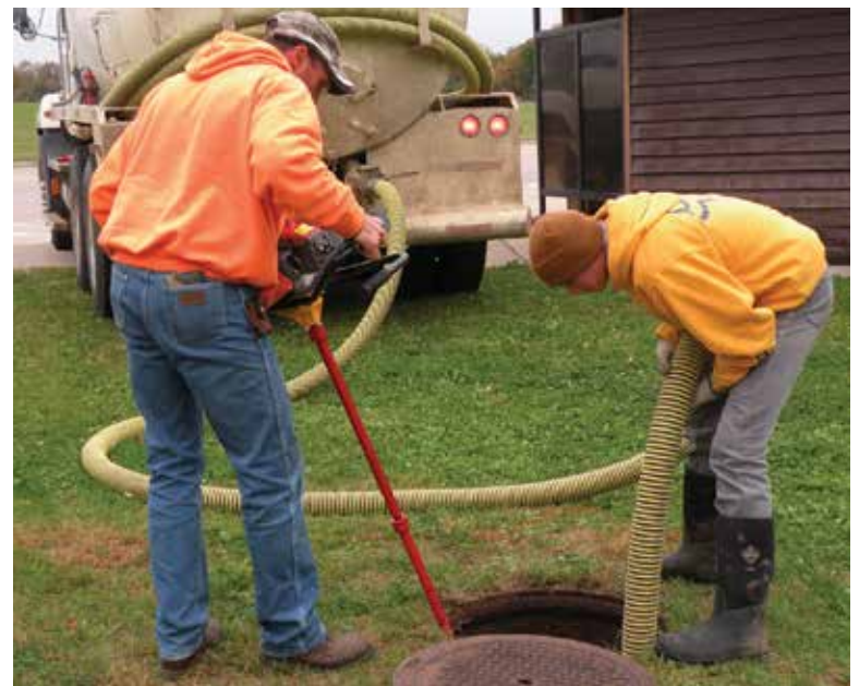
▲ Unidentified septic service workers use a Crust Buster tank agitator during a pumpout at a Minnesota rest stop.
