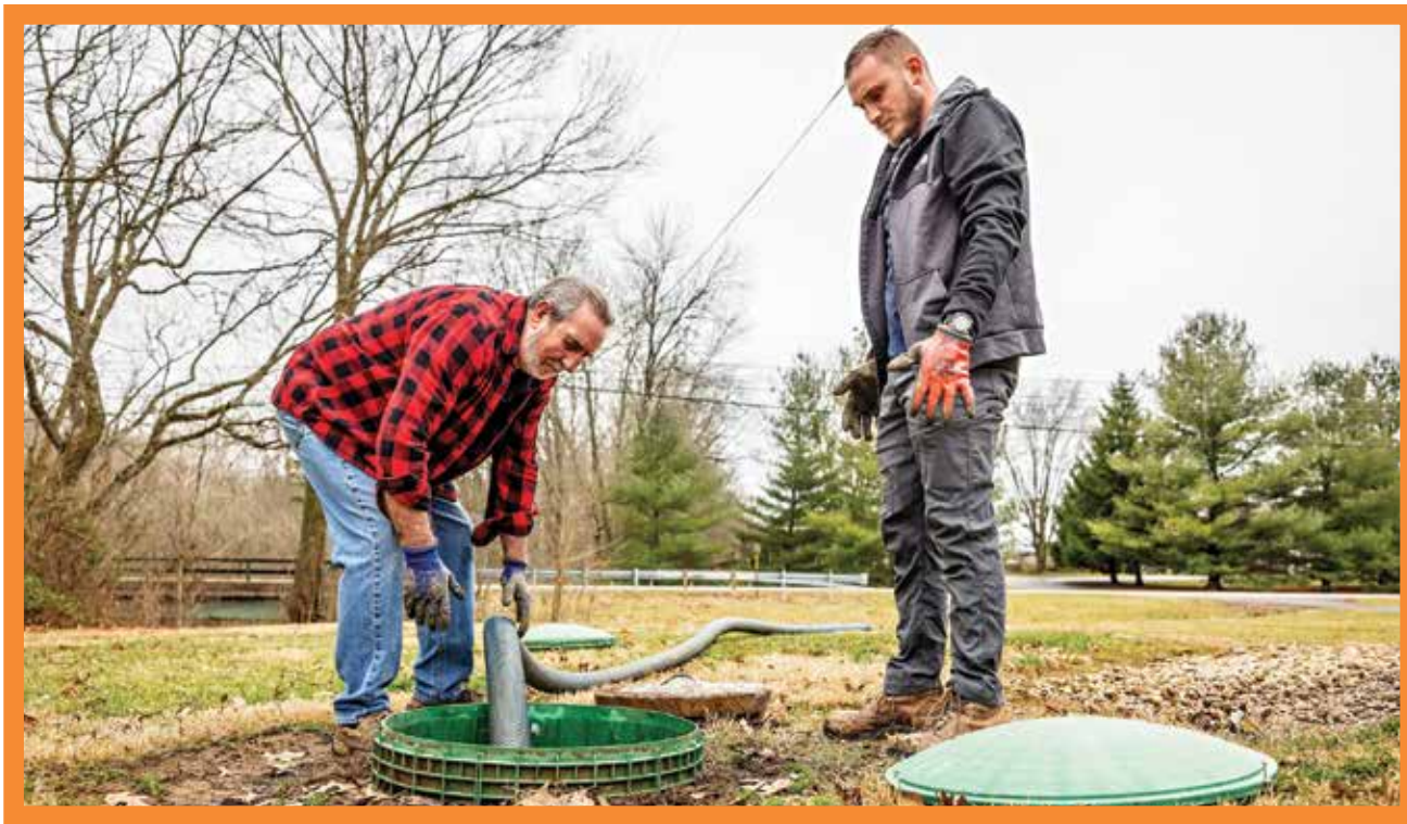
Bill Robinson, left, and Trent Arey perform a pumpout for a residential customer.
