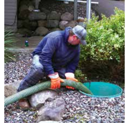
▲ A technician pumps a septic tank.
